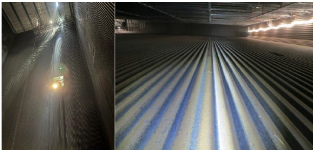
Figure 18. Wall tubes from inside the furnace (internal document from Nilsson, 2023).
