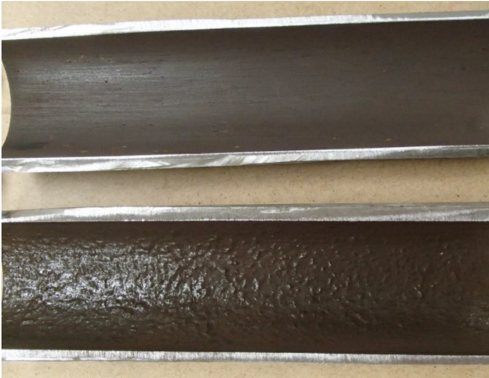
Figure 32. Tube insides after deposits were removed. Cold side (top) is smooth and has minor pitting. Hot side (bottom) has rough irregularities (internal report from Jörgensen, 2018)
