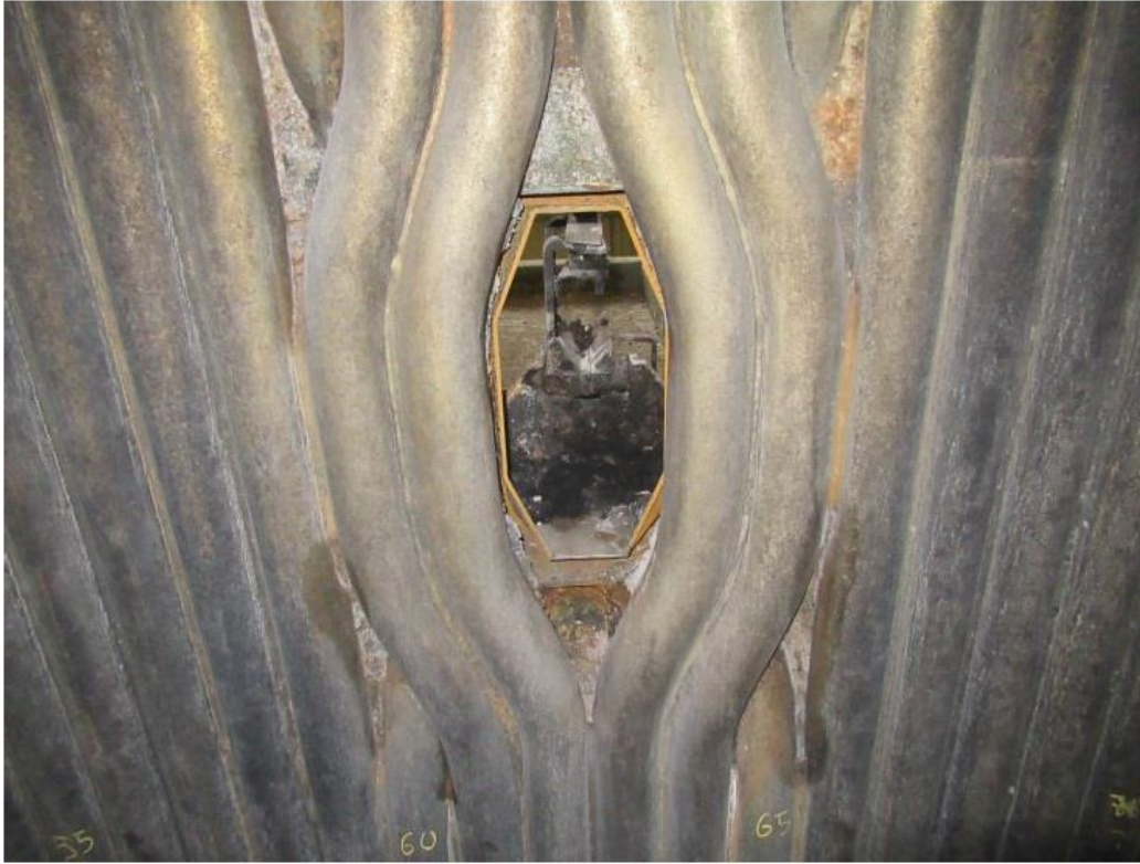
Figure 20. Black liquor gun opening (internal report form Isberg, 2018).
